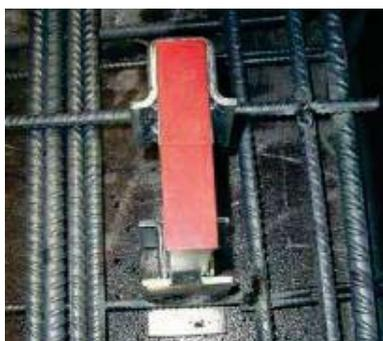
positioning of the Girella bracket insert into a column in phase of arming
