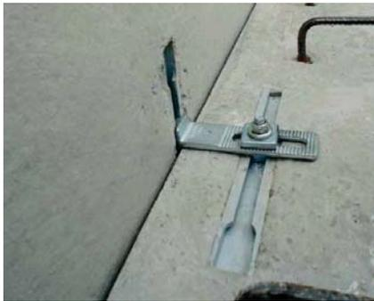
FISIS panel-to-beam shear connection for vertical/horizontal panels
